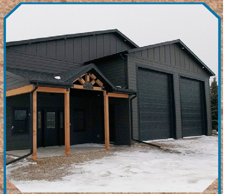
Shop Addition/ Remodeling Project CertainTeed asphalt shingles, and LP Diamond Kote siding with Timber Frame Porch
