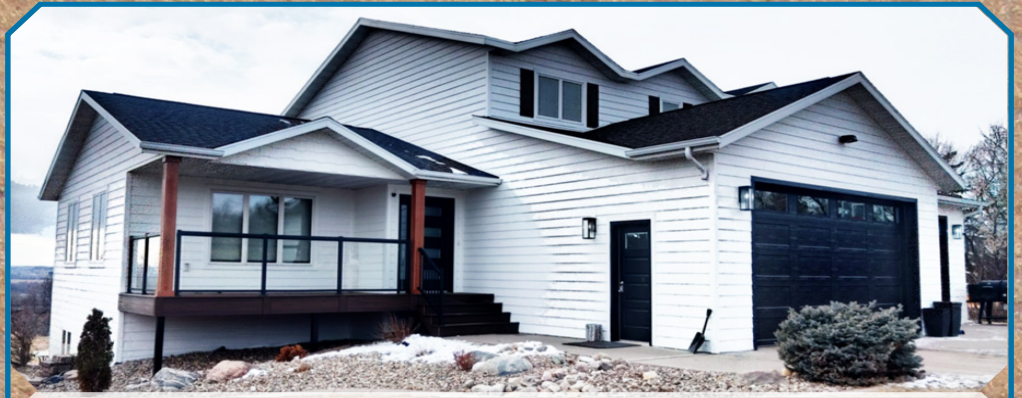
House Remodeling Project CertainTeed asphalt shingles and LP Diamond Kote siding
