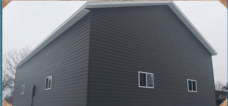
House Remodeling Project CertainTeed asphalt shingles and LP Diamond Kote siding
