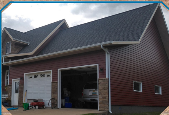
House Remodeling project CertainTeed asphalt shingles, Mastic Steel siding and Versetta on dormers/garage
