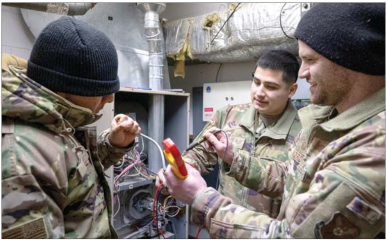
(From left to right) Airman 1st Class Erik Cruz, Staff Sgt. Micheal Villarreal and Master Sgt. Matthew Yordt, all heating, ventilation, air conditioning and refrigeration specialists assigned to the 5th Civil Engineer Squadron, use a voltmeter on an air switch to troubleshoot a furnace at Minot Air Force Base, North Dakota, Feb. 19, 2025. At locations like Minot AFB, where the winters can reach dangerously low temperatures, HVAC/R military and civilian engineers sustain critical heating systems.
