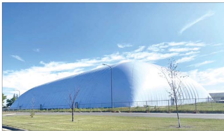
The "Fitness Dome" with the blue turf opened this past fall giving MAFB Airmen and families another place to stay active in the winter months.
