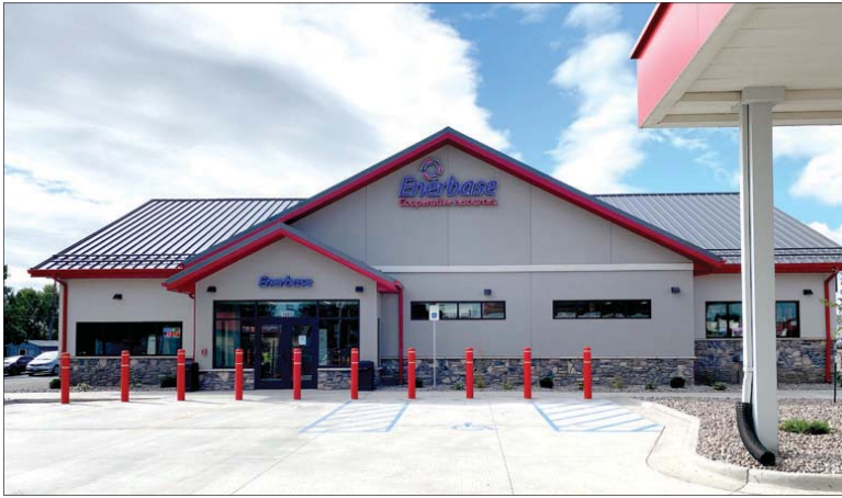
Exterior of new Enerbase Convenience Store
