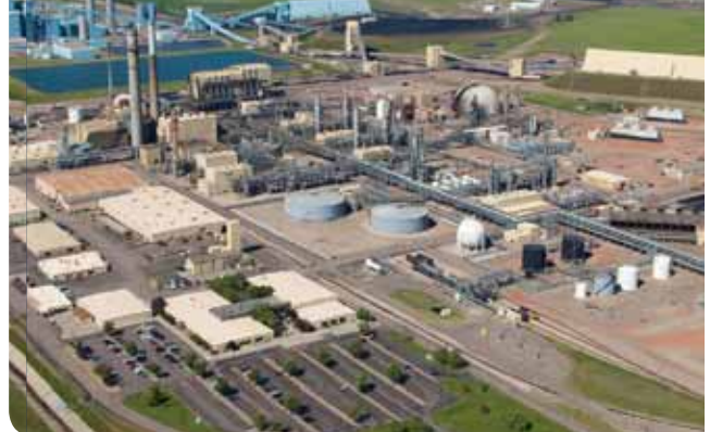
Great Plains Synfuels Plant
