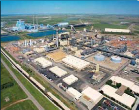
Great Plains Synfuels Plant
