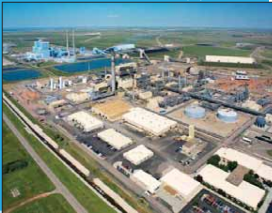
Great Plains Synfuels Plant
