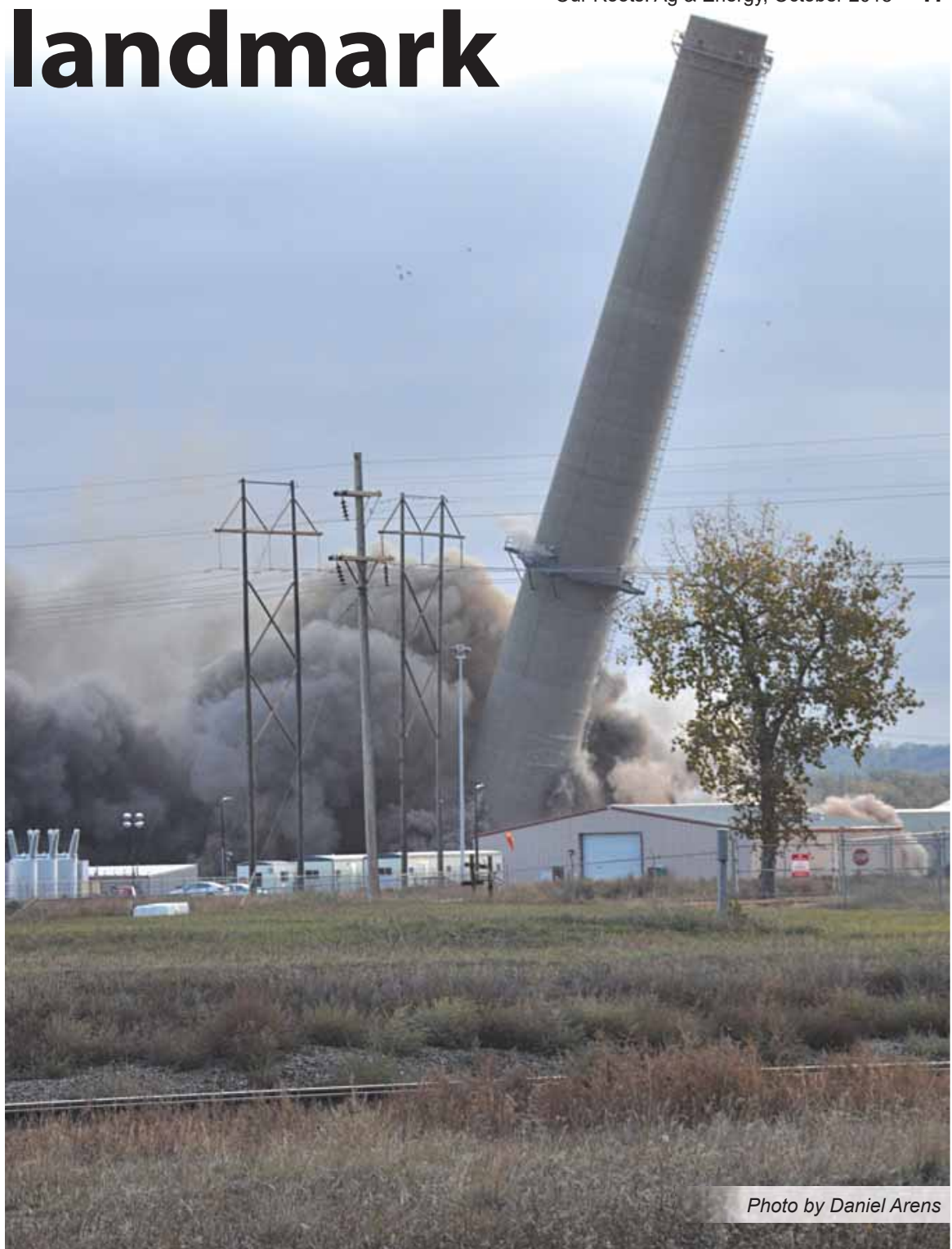
After the detonation of 108 explosion points, the boiler houses of Stanton Station collapse. The demolition, which occurred early in the morning Oct. 11, marks the final chapter for a power plant and Mercer County landmark that was in operation for 50 years.
