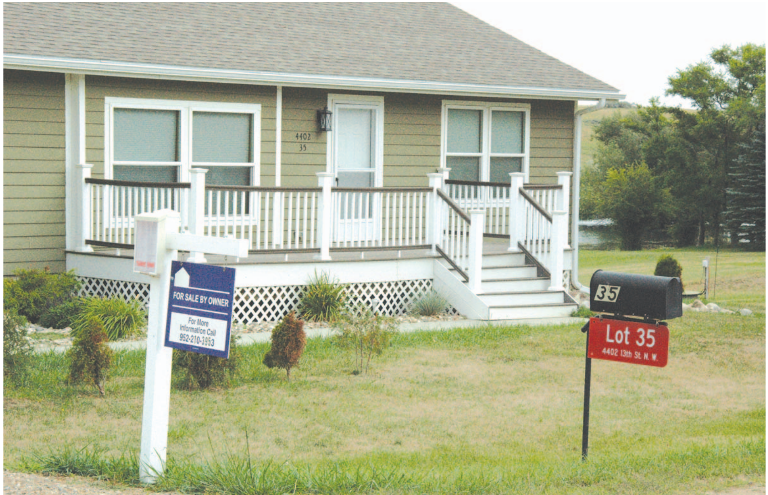
One of the houses currently on the Garrison market. According to realtor Mike Matteson, Garrison has low income housing available through the housing authority and a healthy real estate market overall, but it can be difficult for young professionals to afford starter homes.
