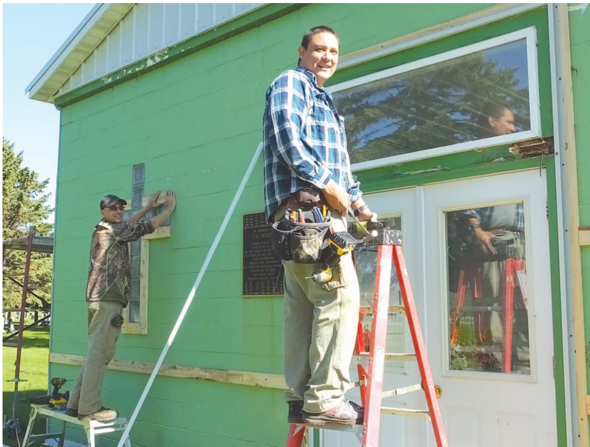
From right, Jake Archambault works on removing the rotted wood over the door while Jesse Rhoads installs the lumber to support the steel siding on the concrete block cemetery building.
