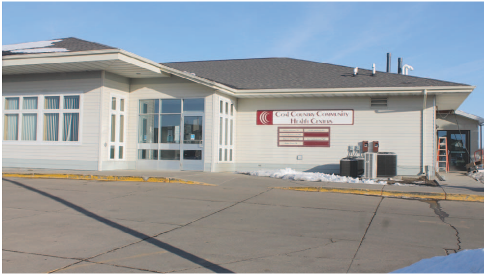
What the clinic looked prior to renovations.
