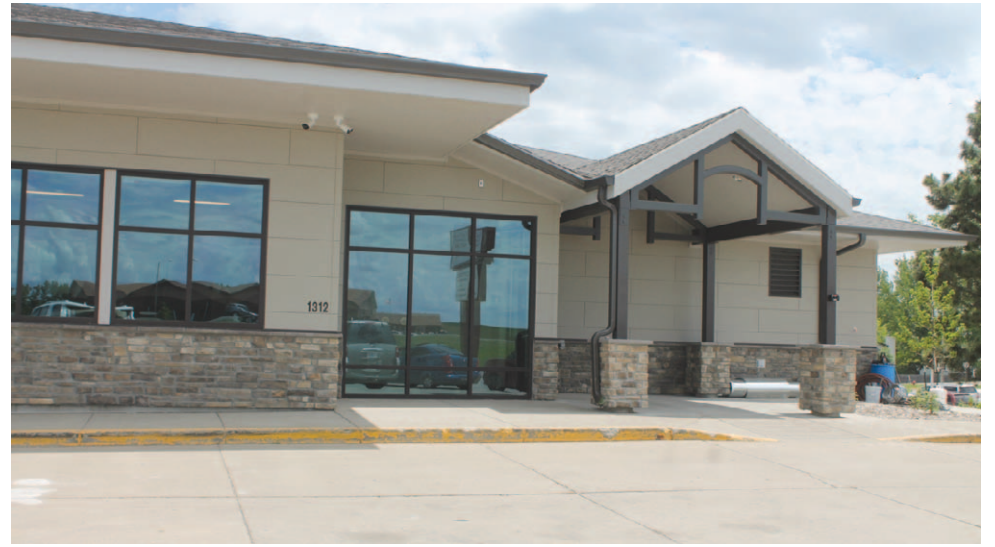
What the exterior of the clinic looks like now.
