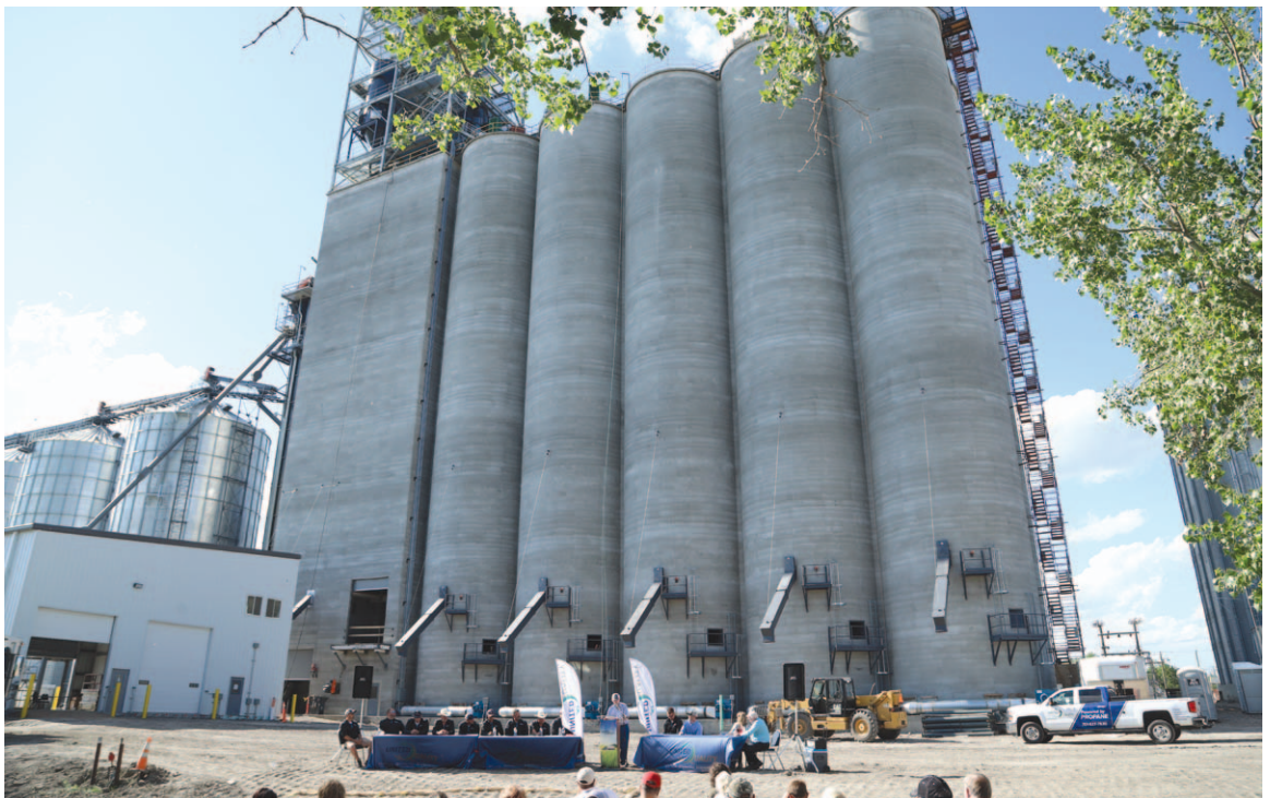
The 150 foot tall bins topped by 120 foot legs of the United Quality Elevator tower over the ceremony marking its dedication on June 27.
