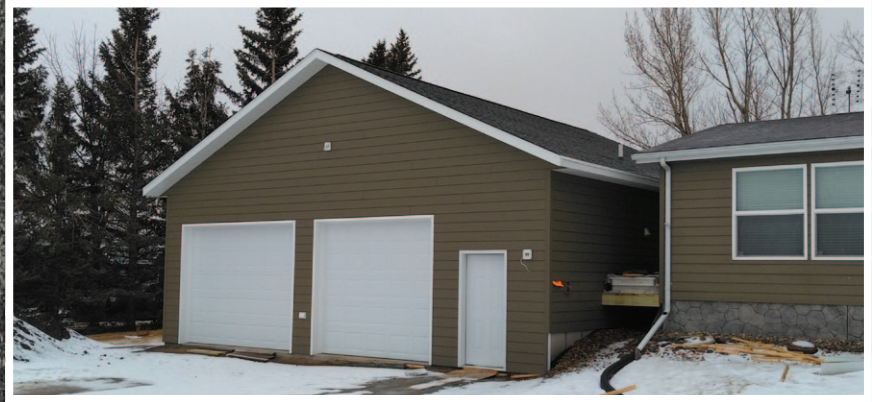
New Garage Construction
