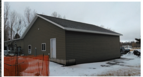
Barn reroof Malarkey asphalt shingles
